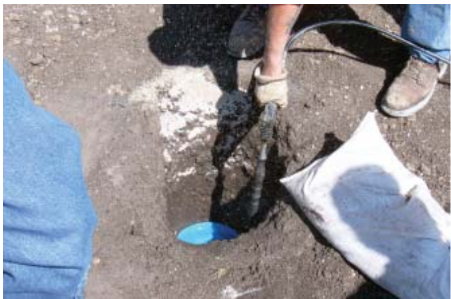
Anode is backfilled with limestone fines, native soil, and water.
