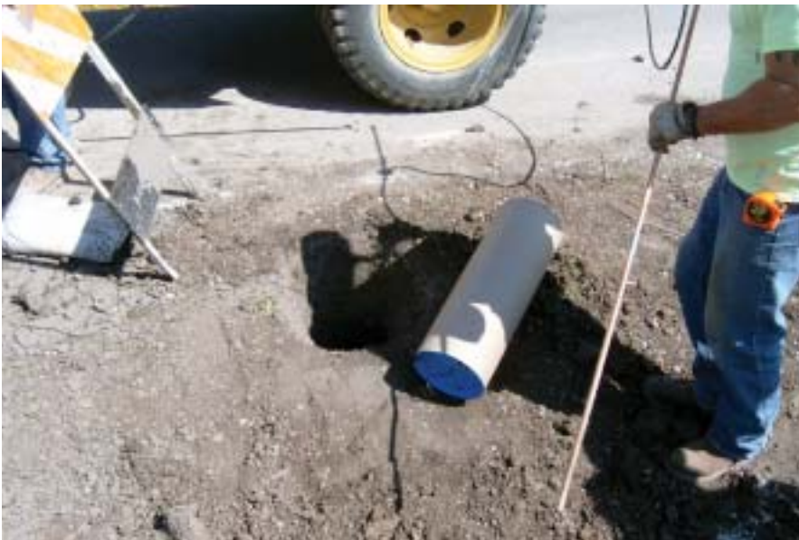
Prepackaged sacrificial anode is lowered down into the hole.
