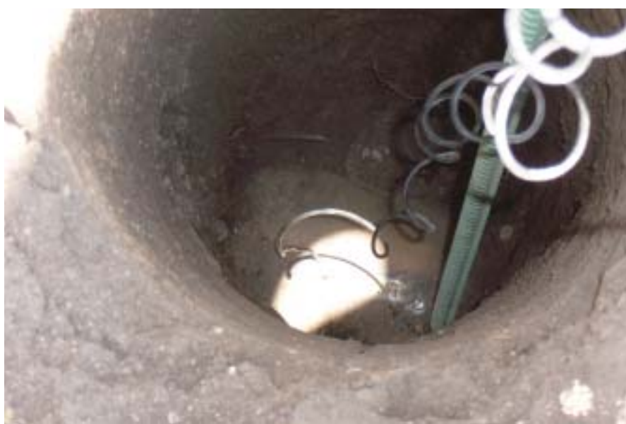
Steel stud arc welded to the top of the pipe.
