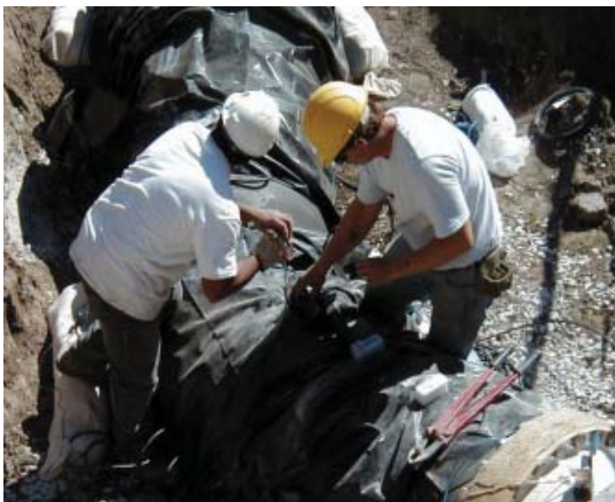
Connecting cable bonds using exothermic welding.
